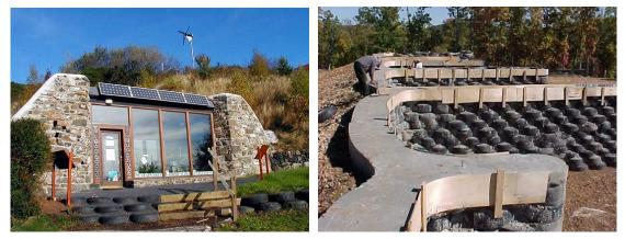
Figure 46. Re-use of old tyres in construction. Source: homedit.com
