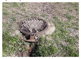
*Figure 6.* A manhole with a local sewerage system for greywater of a school in a rural area. The greywater pipe ends in a ravine, which can be transported to the river by the stormwaters.
