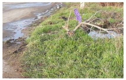
*Figure 3.* Overflow of wastewater from the centralized sewerage system (a village near Chisinau)
