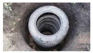
Figure 5. A DIY cesspool made of tyres. Source: decoexpo.com
