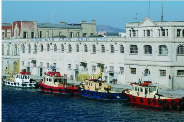
Port Thessaloniki - Passenger Terminal
